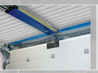
The automatic *CARGO door system* with door operator guarantees easy, safe and reliable opening and closing of the door by pressing a button. If the door operator is not used, it may be easily disconnected from the outside, and the door can then be manually opened and closed without any waiting time.
